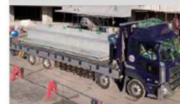
③現場にPCa部材を運搬
