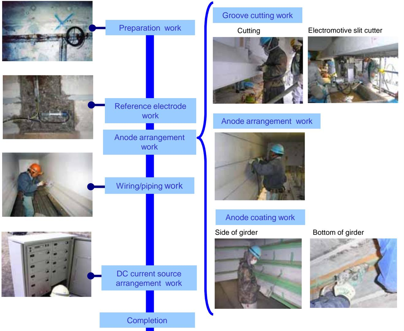
Cathodic protection(PI-Slit method)
