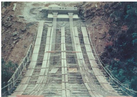
Preliminary Cable Installation
