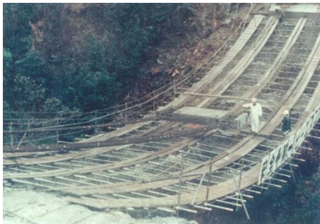
Precast Slab Installation
