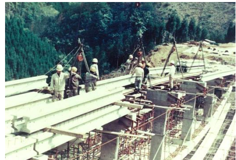
Installation of Stiffening Girder
