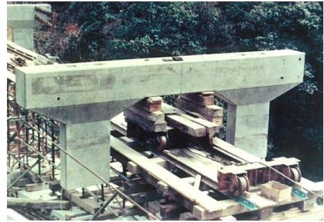
Erection of the Vertical Member
