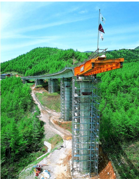
Construction of the Superstructure Through the Launching Nose
