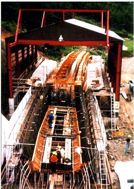
Manufacturing of The Main Girder
