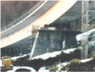
Side Reinforcement for The P7 Pier
