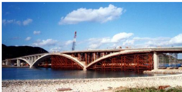
Construction by Scaffolding (Specifically P5)
