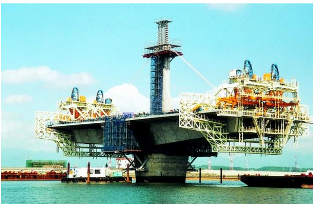
Erection Equipment for Segments
