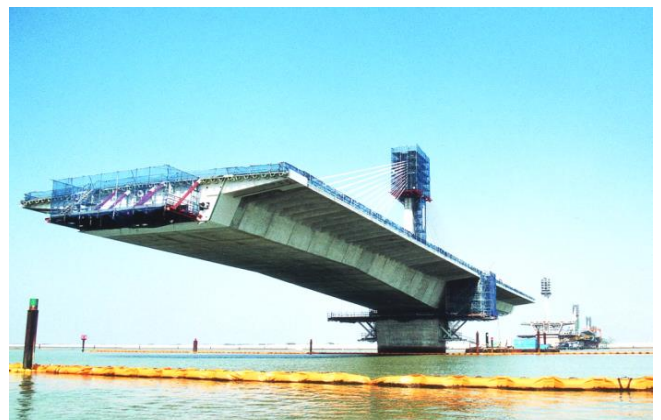
Completion of the Segment Installation
