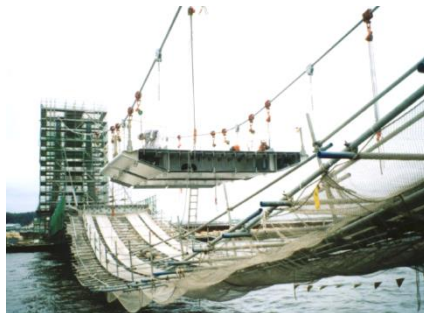
Steel Girder Installation
