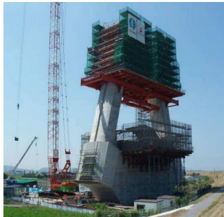
Main Tower Construction by Using The Ascending Formwork
