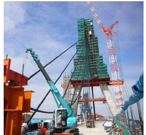
Diagonal Support Installation
