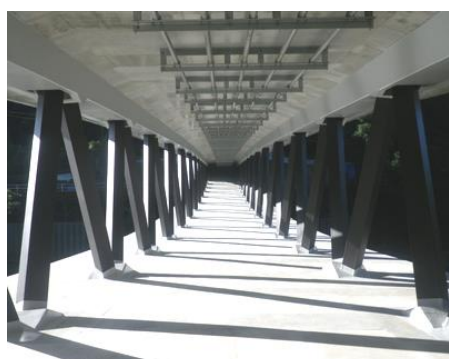
Innert View of The Girder and The Squared Steel Pipe Providing Diagonal Support
