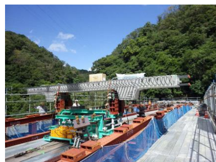
Upper Slab Installation
