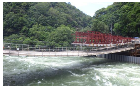
Preliminary Cable Installation
