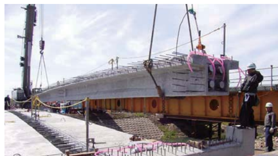
Photo 5 Situation of erection of the girder
