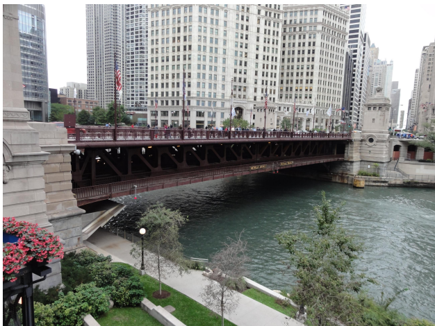
写真-5 Michigan Avenue Bridge
