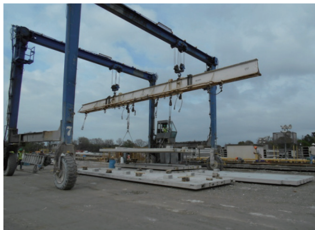
写真-5 East Texas Precast Co.
