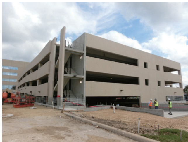
写真-6 Methodist Stone Oak Hospital Parking Garage
