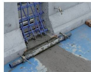
写真-4 間詰め部嵩上げ
