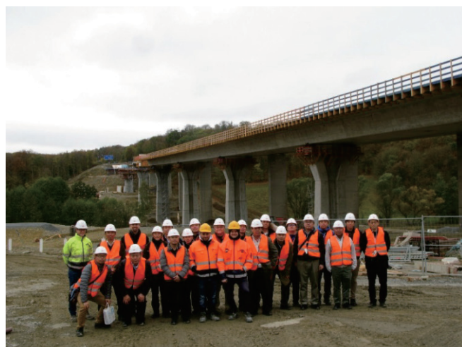
写真-2 Pleichachtal bridge
