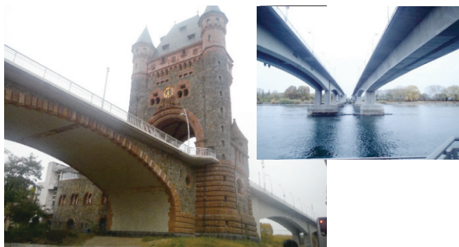
写真-3 Nibelungen bridge
