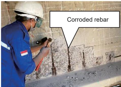
Photo-1 Corrosion damage on PC girder
