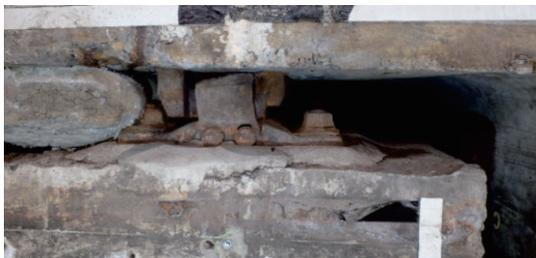
Photo-1 Damaged shoes found in a Gerber hinge
